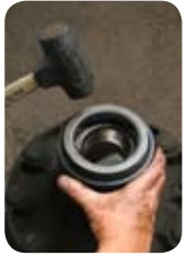
A rubber mallet may be used to tap into place.
